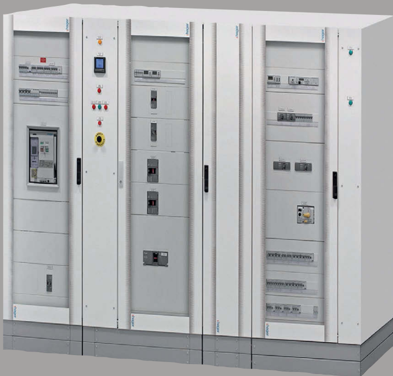
Switchboard for electrical distribution.
